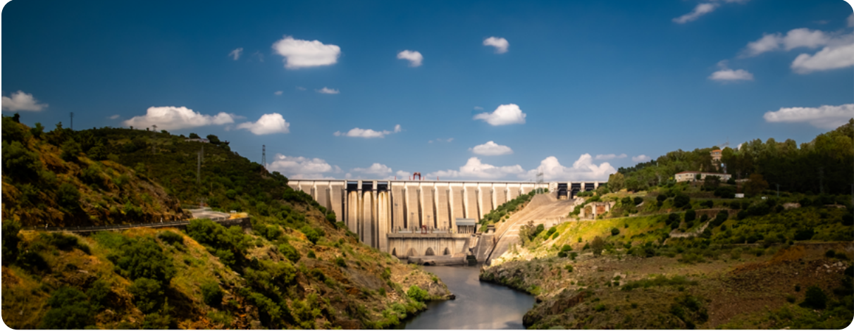
Jose Maria de Oriol hydroelectric power plant, Cáceres, Spain
