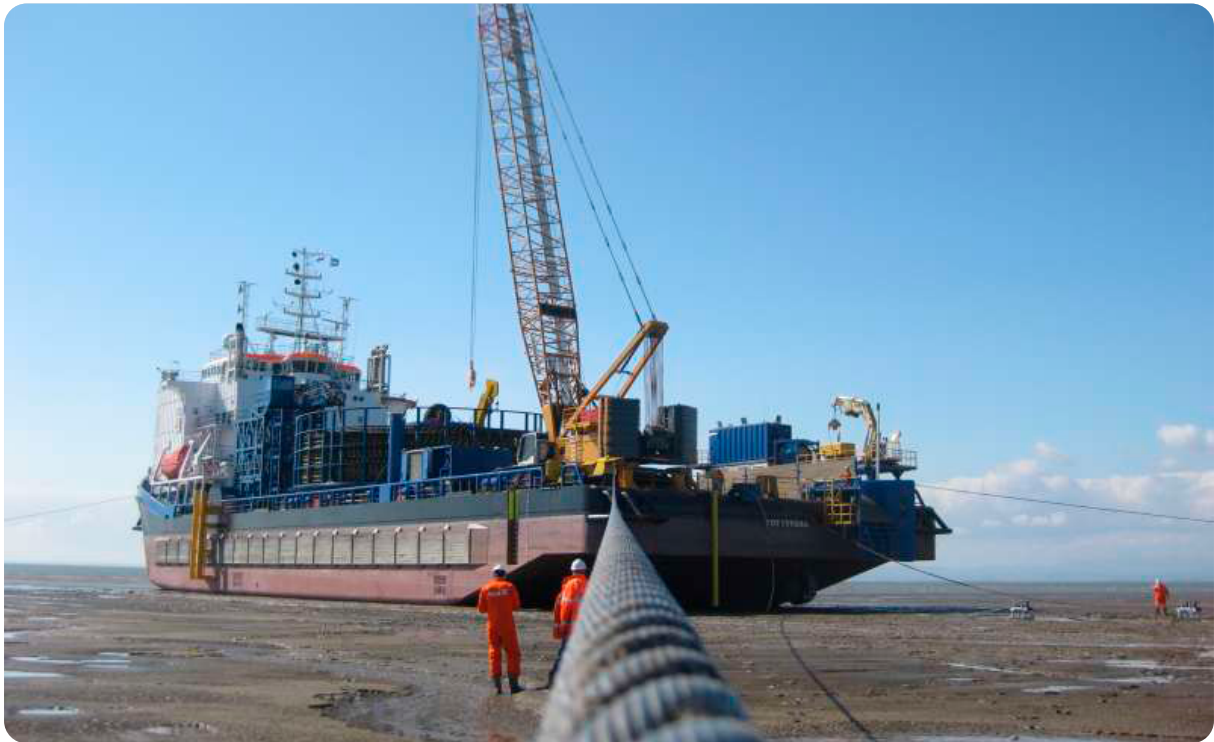
Installation of the Western link submarine cable in Barrow, UK
