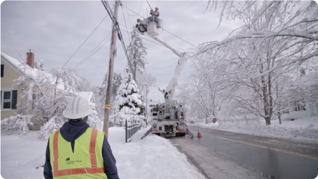
Central Maine Power (Avangrid) workers restoring electricity service in Maine, US.
